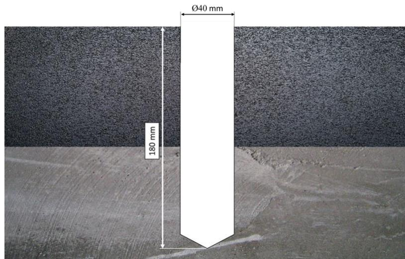
**Figure 2:** Dimensions of the opening for Parking pill
